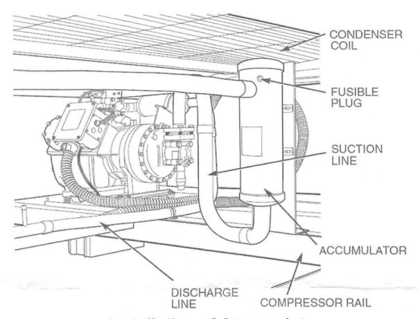
Installation of Accumulator 38AK500410 Shown
